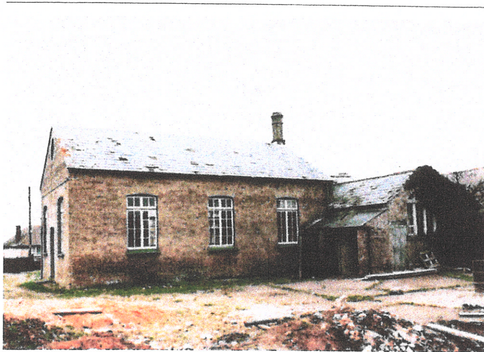
View of the back of the chapel and school. The school is the small building on the right of the picture.
